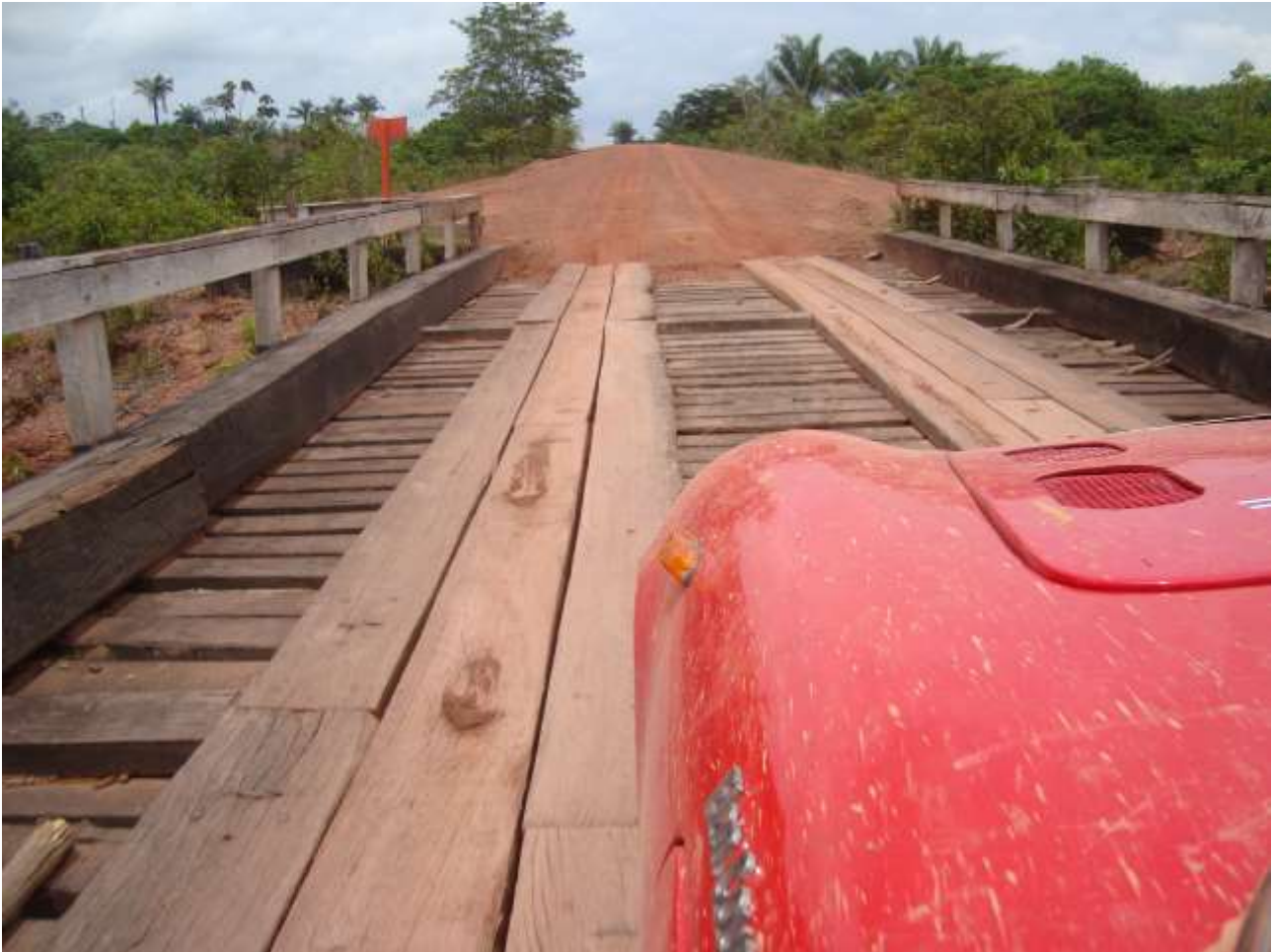
Transamazonica highway bridge
